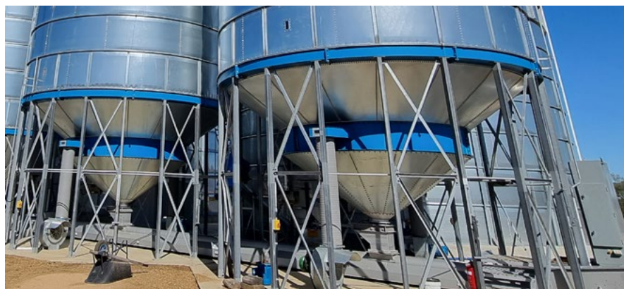
Photo 2: A purpose-built silo for aeration drying has a large fan capable of more than 15L/s/t with ducting right around the silo cone. (Source: Alex Conway)
