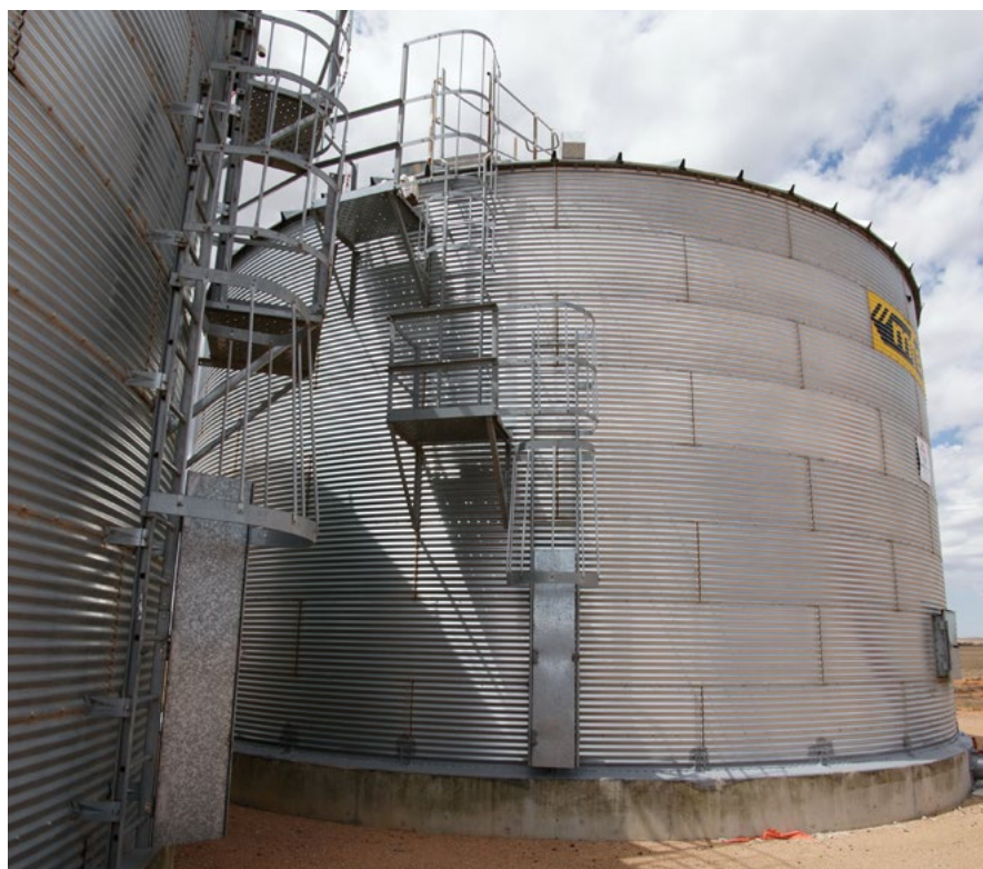
Photo 5: Caged and platformed access ladders improve safety when climbing the silo to inspect stored grain. (Source: Ben White, Kondinin Group)
