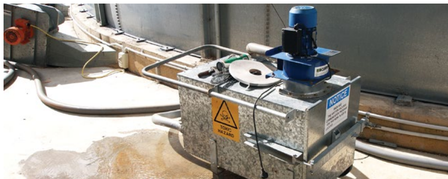
Photo 10: Powered recirculation improves gas distribution through the silo enabling 7-10 day exposure rather than 20 day exposure when fumigating silos greater than 300t capacity. (Source: Chris Warrick, Primary Business)
