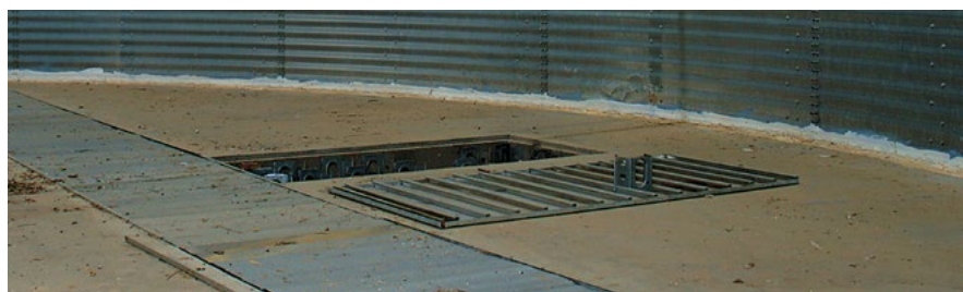
Photo 6: In-floor aeration ducting in flat-bottom silos, which can be removed for cleaning, is ideal. (Source: Ben White, Kondinin Group)
