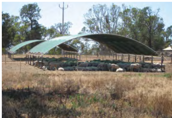
Another view of the shade structure. Photo Credit: Geoff Duddy.
