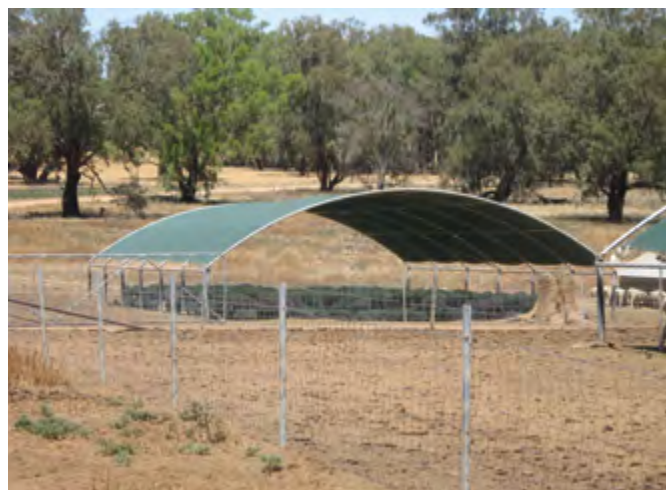
Sheep under shade in a feeding area. This shade allows for airflow through and about. Will have some areas that will not get the sun and may not dry out. This could be an issue for cattle. Photo Credit: Geoff Duddy.
