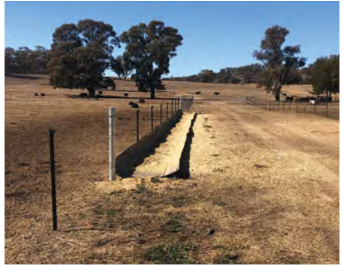
Well planned feeding area, however this area lacks slope in some locations and has a flow line running through it. Photo credit: Brett Littler.
