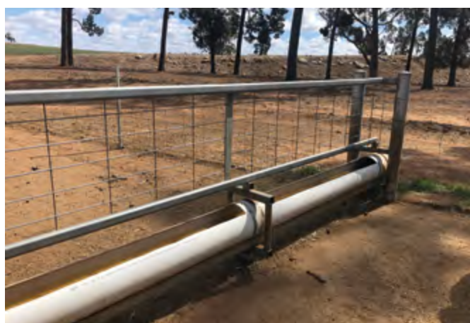
Another view of the PVC pipe trough. Note how this trough when cleaned drains out into the paddock and not into the pen. Photo Credit: Sue Street.
